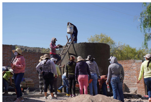
Photo: A group of community members from La Norita del Refugio building a Rainwater Harvesting System.
